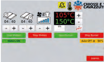
Griff PLC interface
